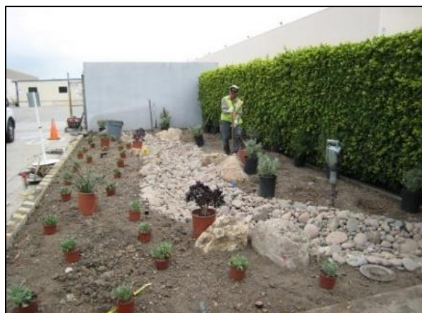
Bioswale construction and establishment.
